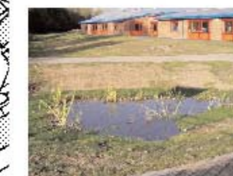
WET PONDS are basins that have a permanent pool of water. They provide temporary storage for additional storm runoff above the permanent water level.
