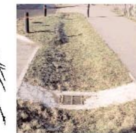
SWALES are broad, shallow channels covered by grass or other suitable vegetation. They are designed to convey and/or store runoff, and can infiltrate the water into the ground (if ground conditions allow).
