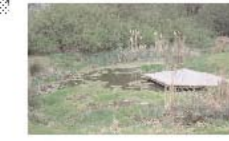
CONSTRUCTED WETLANDS are ponds with shallow areas and wetland vegetation to improve pollutant removal and enhance wildlife habitat. These are regarded as one of the most effective SUDS techniques for biodiversity and water quality improvements.
