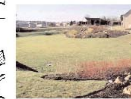
EXTENDED DETENTION BASINS are normally dry, though they may have small permanent pools at the inlet and outlet. They are designed to detain a certain volume of runoff as well as providing water quality treatment.
