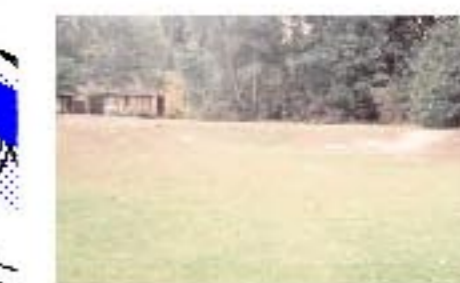
INFILTRATION BASINS are depressions in the surface that are designed to store runoff and infiltrate the water to the ground. They may also be landscaped to provide aesthetic and amenity value.
